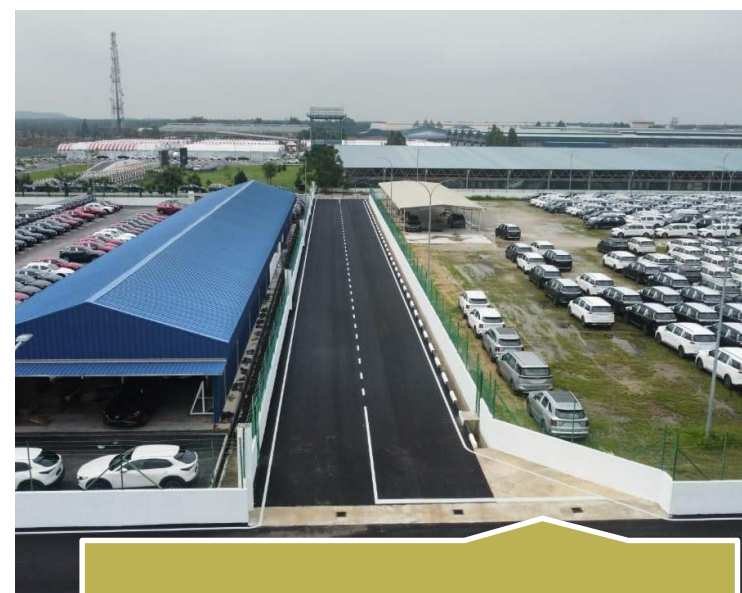
Crusher Run Parking
